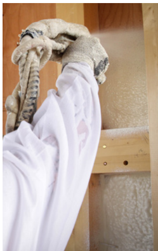
Open Cell Wall Foam Application
