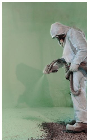
Under slab application with Closed Cell HFO Spray Foam (Radon protection)
