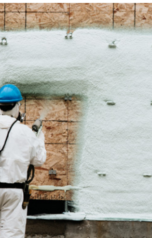
Exterior Continuous Insulation with Closed Cell HFO Spray Foam
