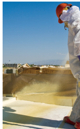
Roofing Foam Application
