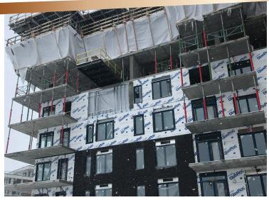
Example of productivity of the D-Max system. The cladding is installed from the ground floor to the third floor, the interior insulation is installed on levels 4 and 5 and the structure is poured on levels 6 and 7
