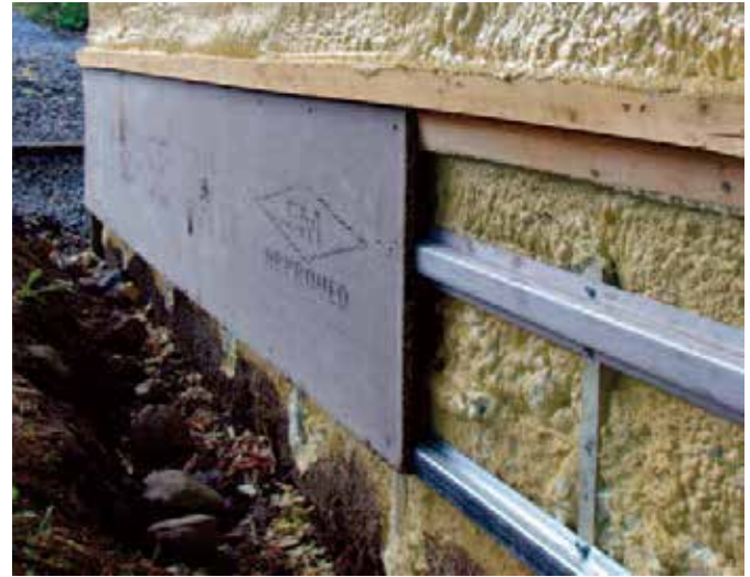
Example of the above-grade portion of the foundation during construction.
