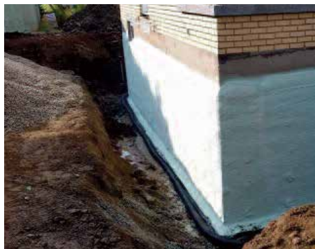
Heatlok HFO is ideal for insulating old concrete or stone foundations from the exterior.
