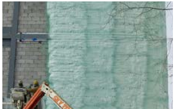
Heatlok HFO being installed directly on CMU block from the exterior.
