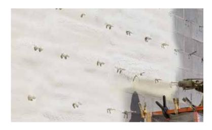
New advanced closed-cell, medium-density spray foam insulation. Huntsman Building Solutions ProSeal® sets a new benchmark in sprayability and performance. ProSeal offers a higher R-value and improved yield to meet today's strict building code requirements making it ideal for commercial applications. This low VOC spray foam insulation product allows for a higher initial pass of four inches to achieve R-27 as well as a Class II Vapor Retarder in one pass.
