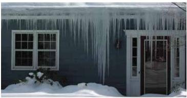
Roofs like these are frequently the source of problems, inside the structure and in the materials. The cause is often inadequate insulation and/or a discontinuity in the air barrier system.
