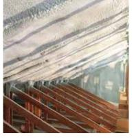
If you want a conditioned attic to use for storage, to install mechanical ventilation systems, or even to turn your attic into a living space, closed-cell spray foam can be sprayed directly onto the roof deck, with no venting. The soffits will have to be sealed and the attic can then be conditioned and will be completely sealed from the outside air. The same concept can be applied to a flat roof. Venting between closed-cell spray foam and the plywood sheathing is optional.
