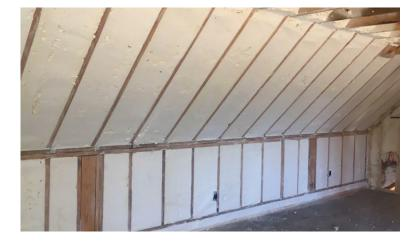
FOAM-LOK 500 is an open-cell spray foam insulation technology that is installed in interior spaces with no ignition barrier required.
