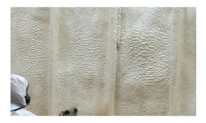
Gain the competitive edge with Huntsman Building Solutions' newest closed-cell spray foam innovation - ProSeal LE - by achieving R-35 in one pass! Suitable for use in commercial and residential applications, this high-performance, low VOC medium density spray foam insulation allows for an initial 5" pass to meet today's stringent building code requirements.
